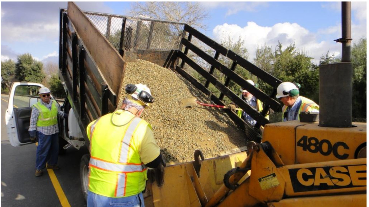
Clem operates the truck's dump-be lift control as Mike F., Frank, and Chris shovel rock into the bucket of the back-hoe
