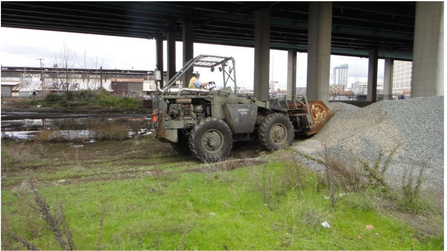
Chris operating Big Green, scoops up more rock for round two of Operation Fair Footing...
