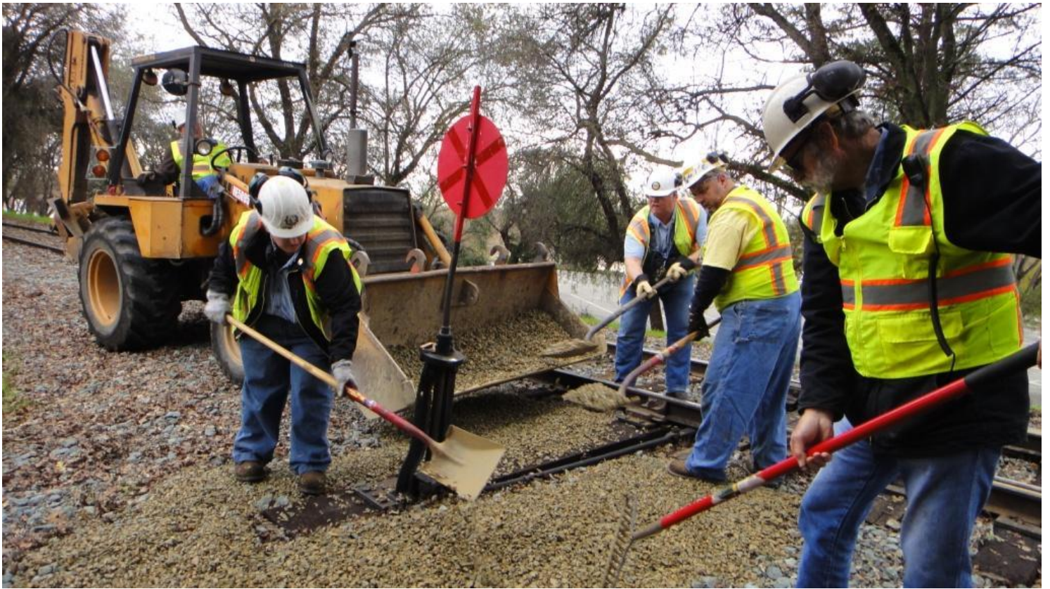
At Switch 16 (south Miller Park) Heather, Chris, Mike F., and Alan create smooth footing around the switch stand
