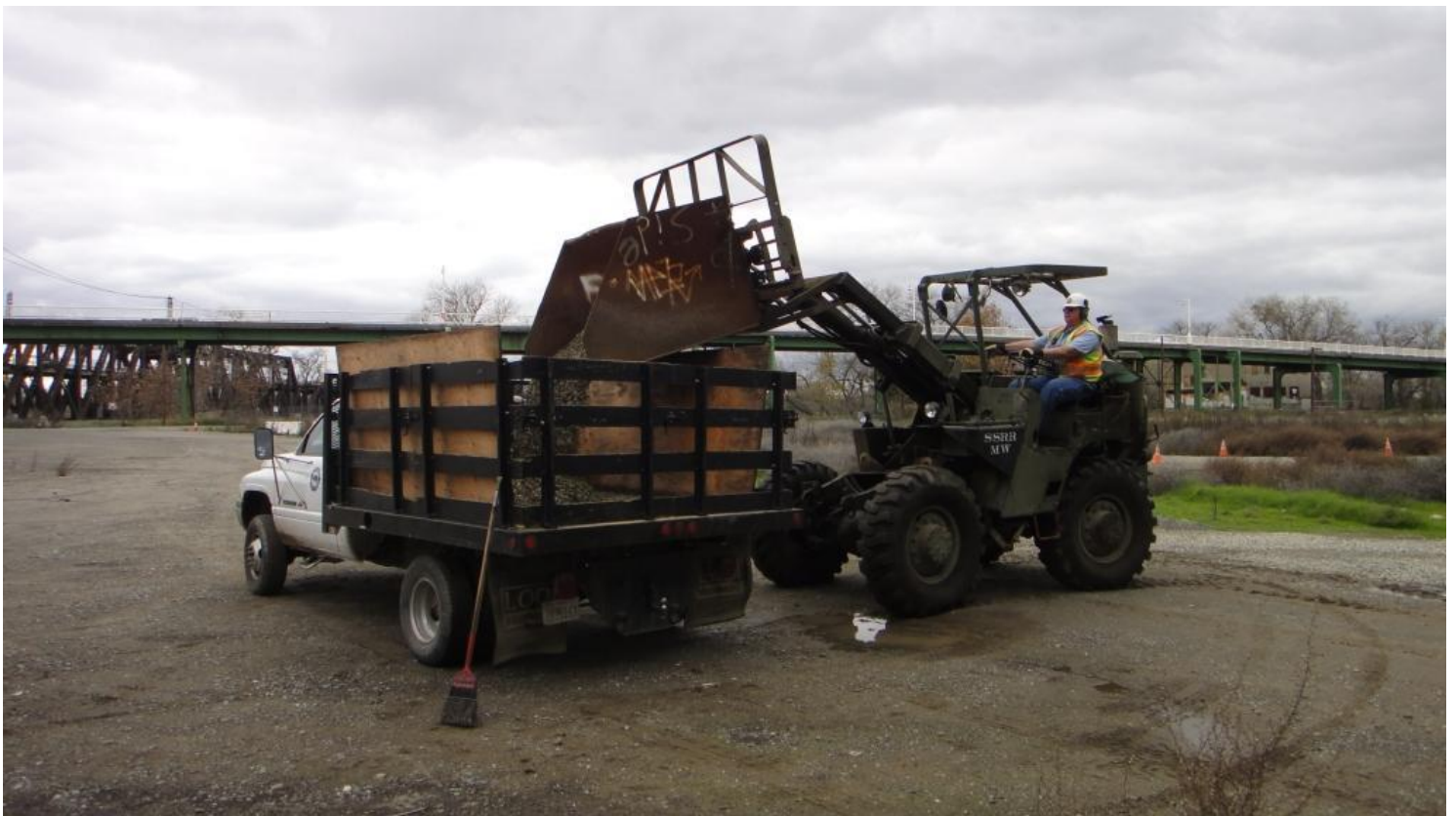
The rock is dumped into the bed of Truck 14
