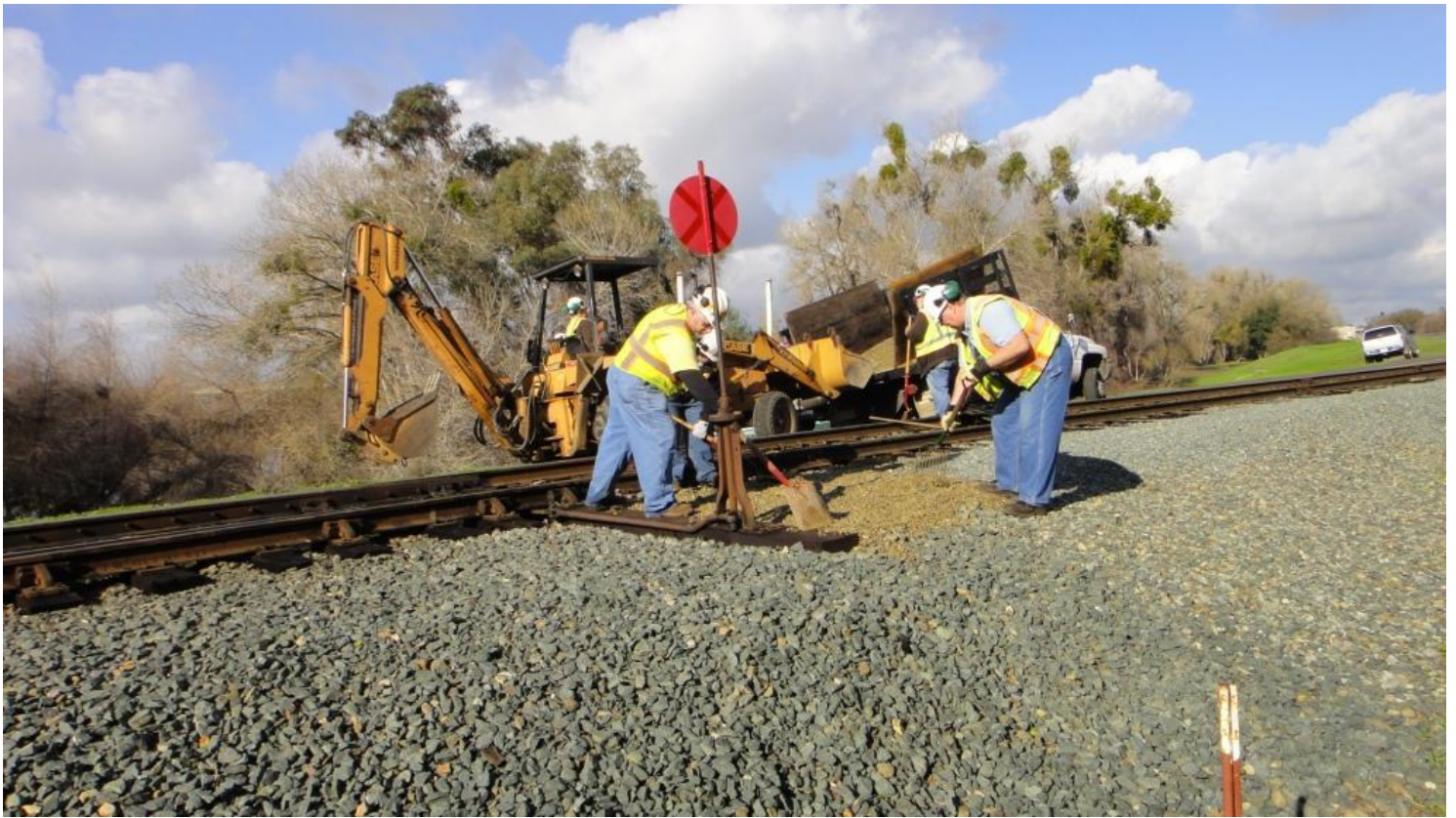
At Switch 17 (north Baths) new footing was installed.
